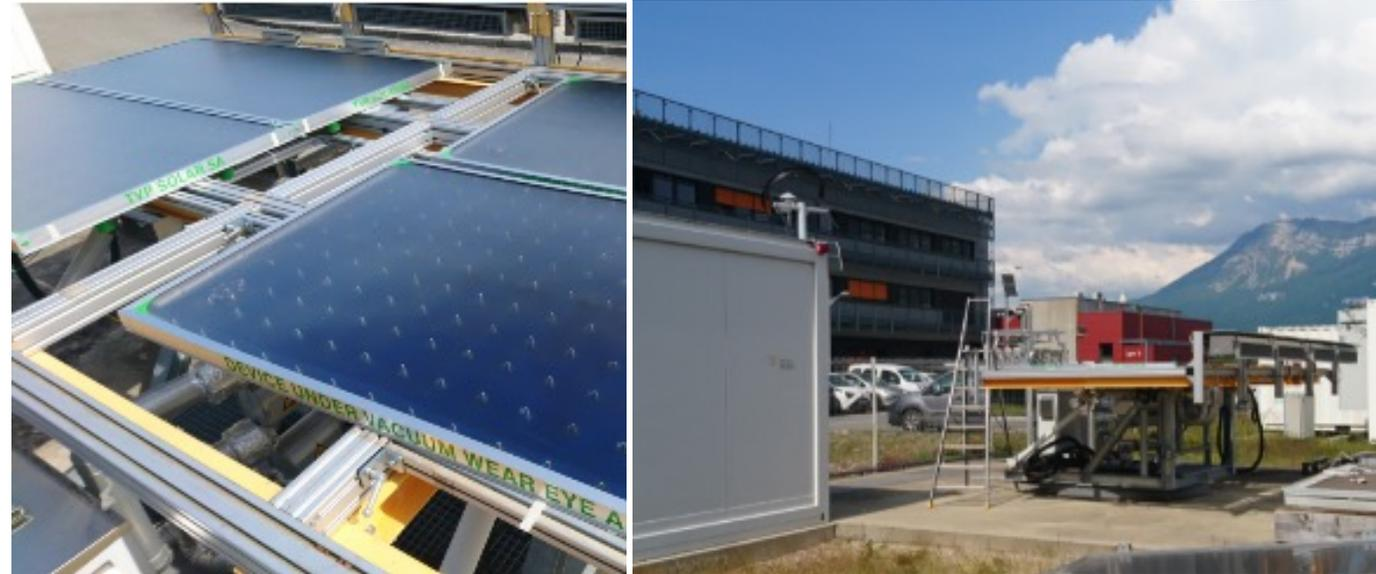
The Sunhorizon demo pilots of **TP3** in Sant Cugat, **TPI** in Verviers and Berlin are relying on **TVP solar LT power high vacuum flat solar thermal panels**.
